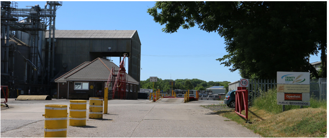
Large scale grain storage at Trinity Grain illustrating strong presence of height and massing; 24 silos and associated infrastructure
