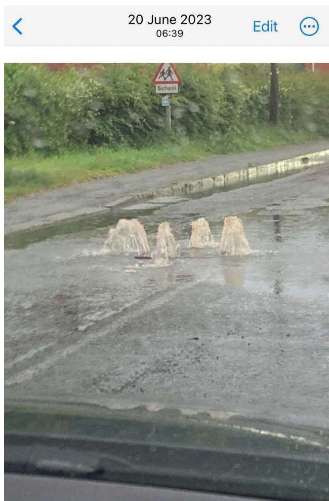
Figure 7. Newbury Street, 20th June 2023
