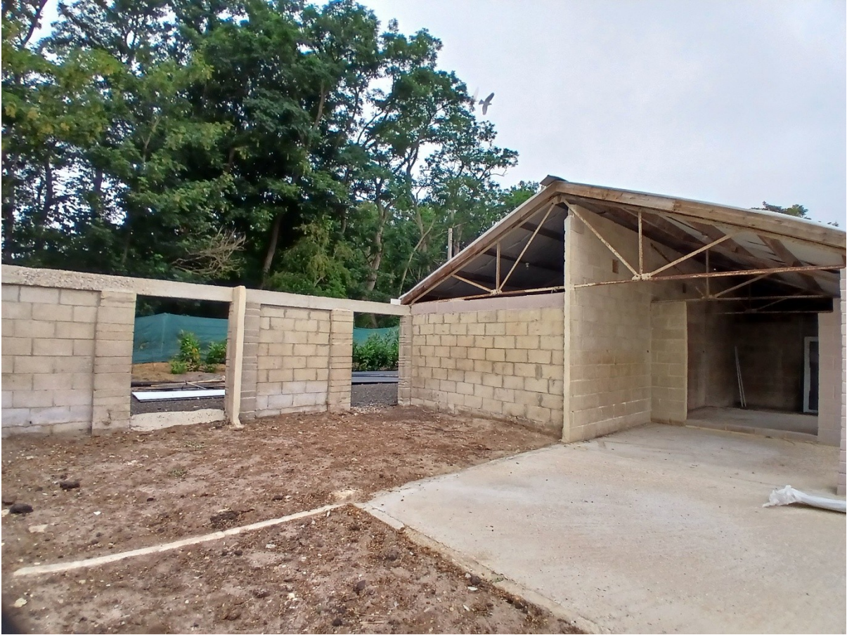
Figure 6: Demolished area with remaining stable openings.
