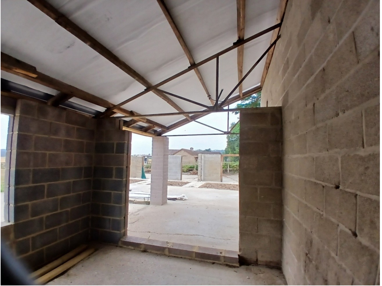
Figure 8: View from inside the incomplete dwelling extension.
