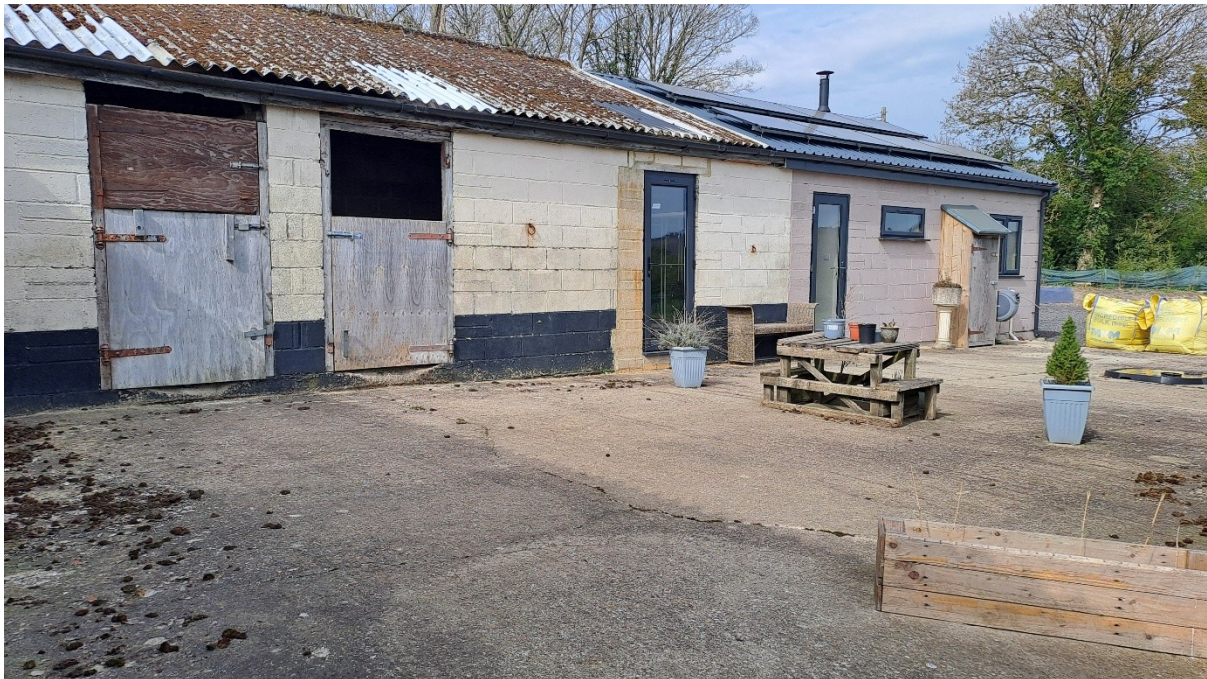
Figure 1: View of northern portion of the L-shaped block with the courtyard in the foreground.
