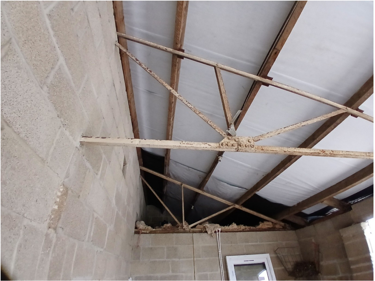
Figure 9: Roof structure. New roofing material.
