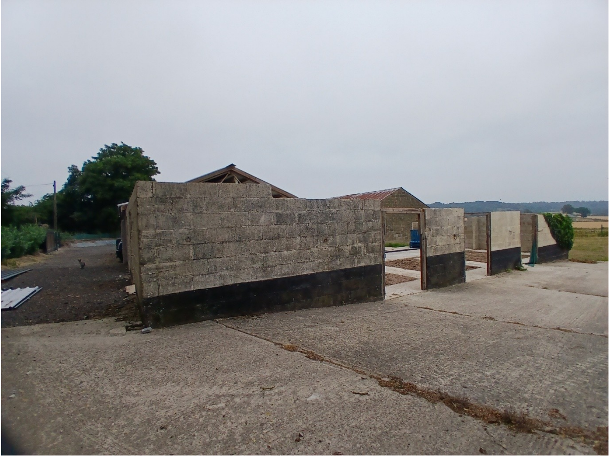
Figure 11: Remaining walls of the southwestern elevation of the former L-shaped building.
