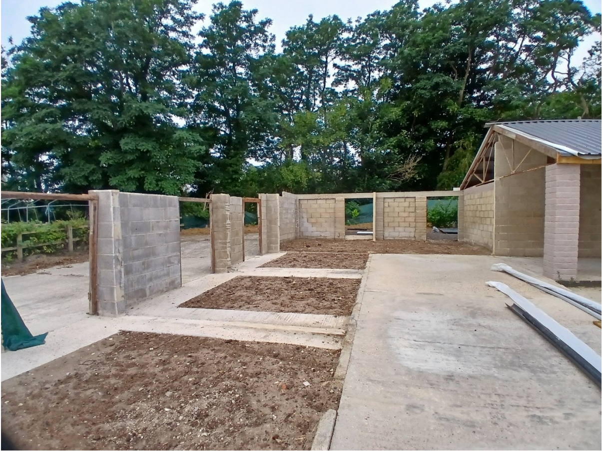
Figure 5: Demolished portion of the building and outer walls with stable openings.
