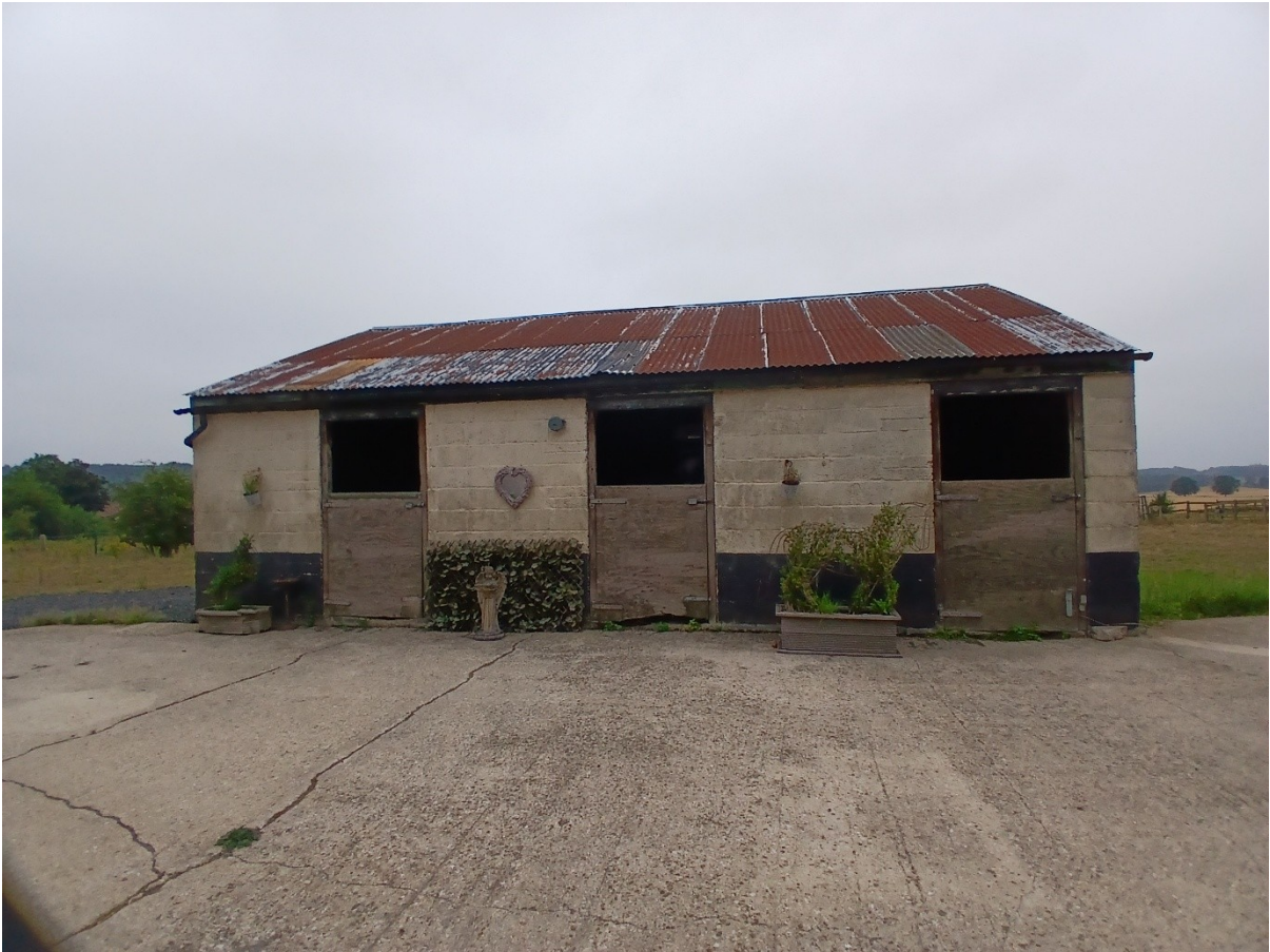
Figure 14: Northern elevation of the southern stable block.
