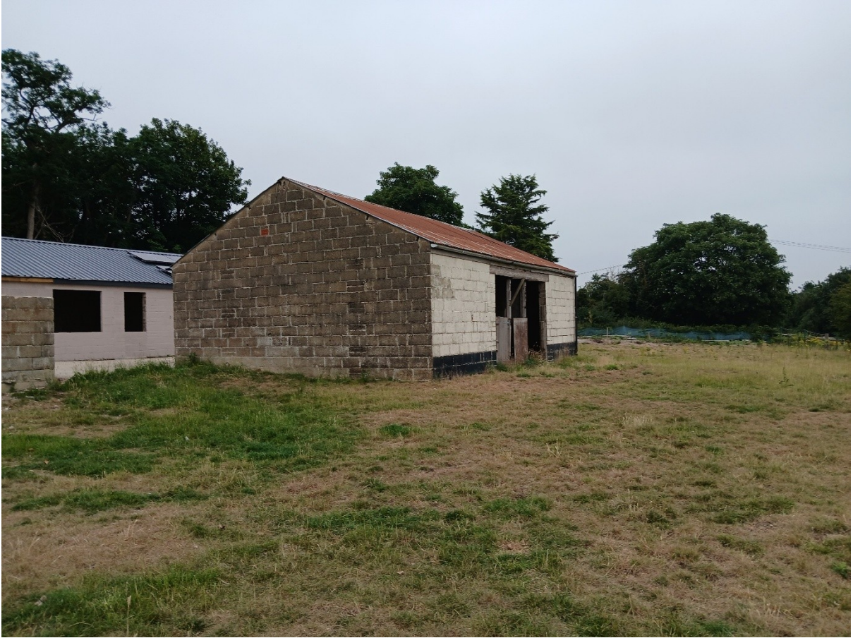
Figure 13: Southern elevation of the southern stable block.
