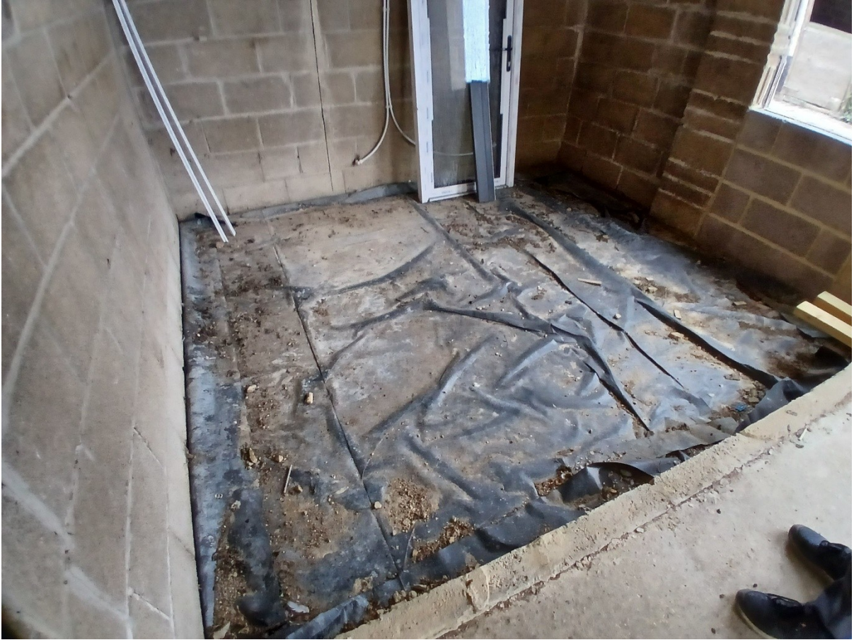
Figure 10: New floor under construction.
