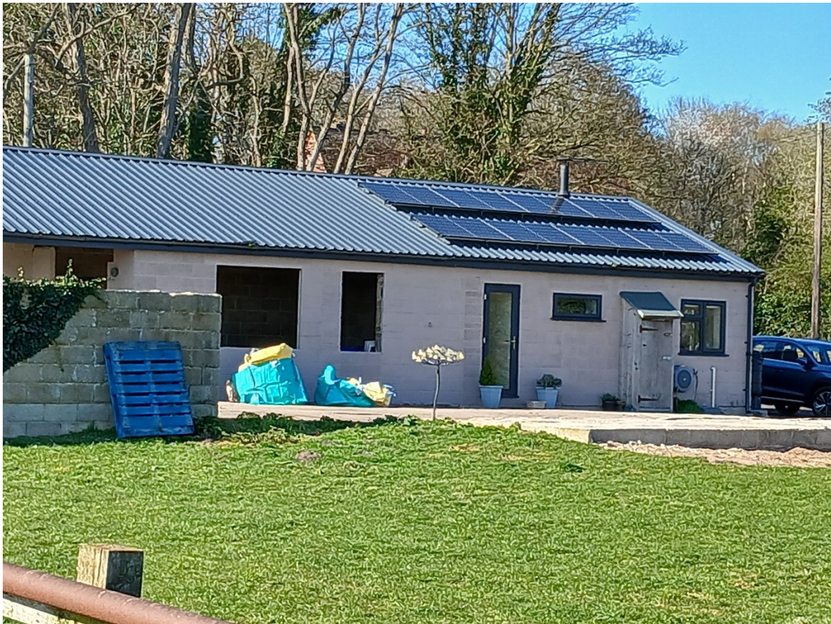
Figure 1: Southeast elevation of the former L-shaped building (by-way behind) and access to the right of this photograph. Southern stable block demolished. The original stable doors have been bricked up and new window openings created (still under construction). Photograph taken from "Solo Chase" (western neighbour) by the Planning Officer.
