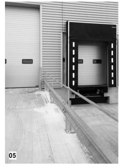
05 DOCK APRON RETAINING WALL External retaining walls to the sides of the dock access will be also of fair faced concrete. Armco barrier galvanised mild steel and handrailing is to be provided adjacent to the retaining wall to level access ramps. The barrier uprights are to be surface fixed to the concrete.
