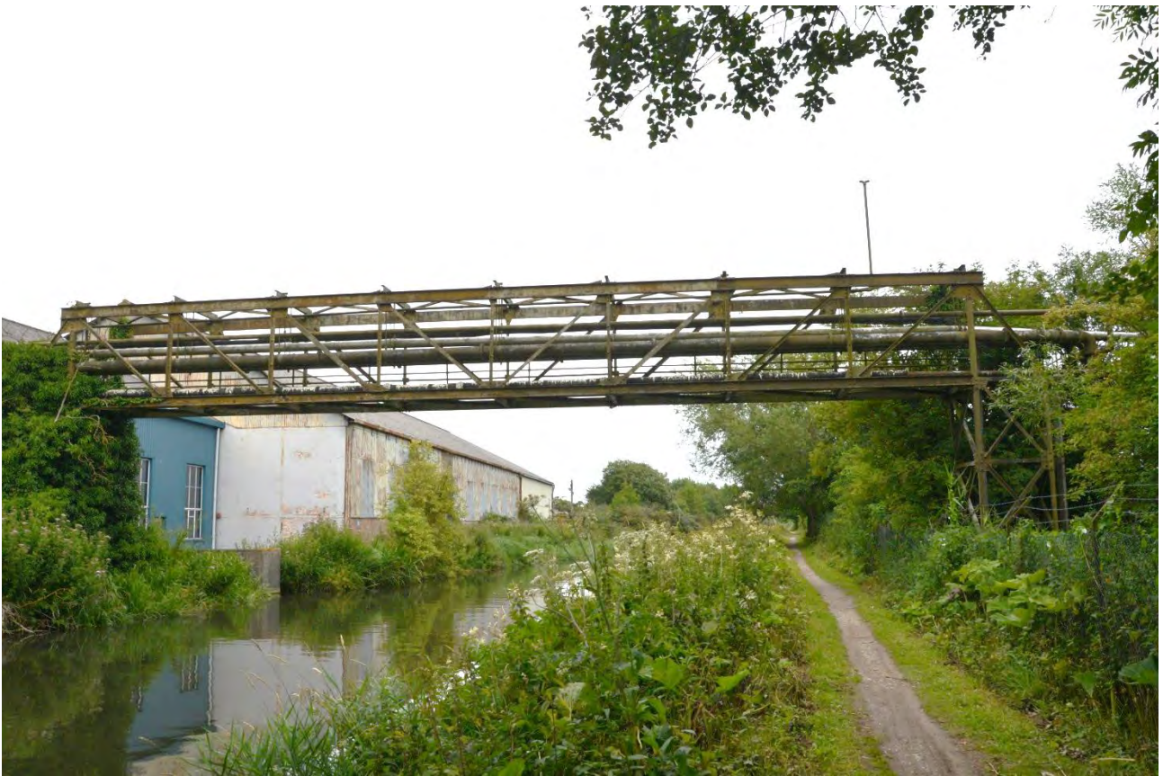
Plate 50: Pipe bridge crossing the canal to area 8
