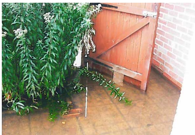
Figure 1 – External flooding at 44 Bartlemy Road
