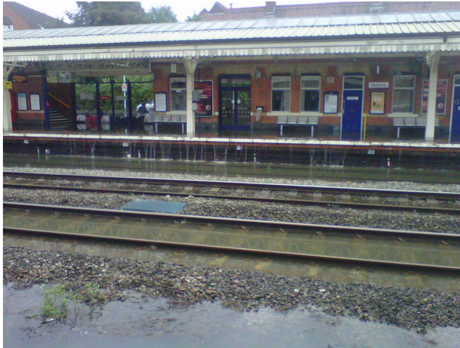
Figure 5 – Train Station and track flooding. Water flowing over the platform
