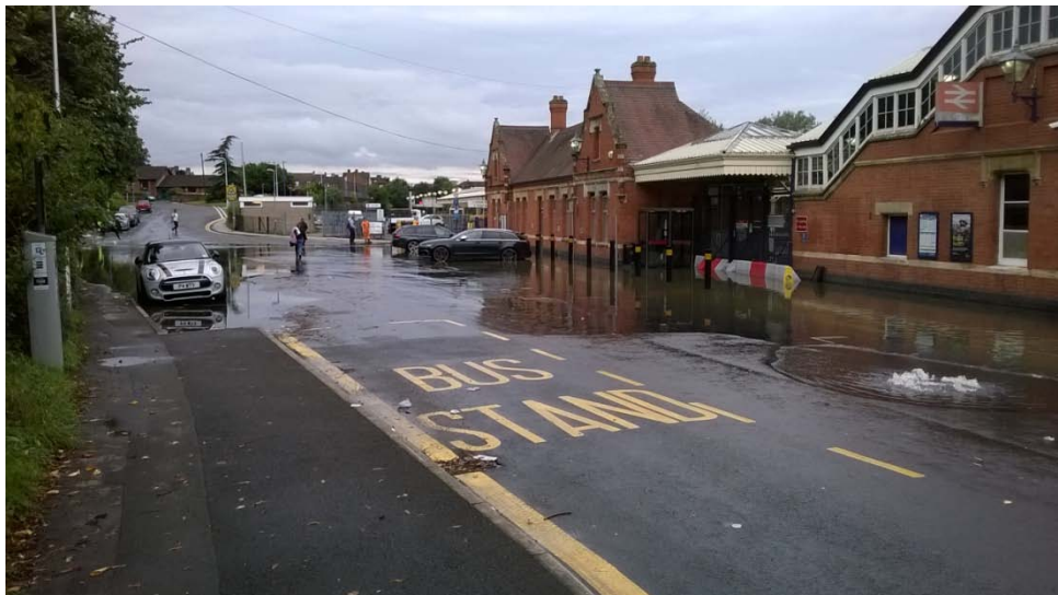
Figure 4 – Flooding of Station Road and foul manhole flooding
