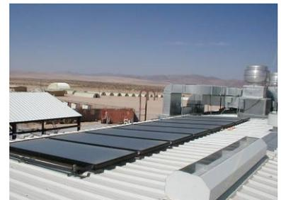
SHW systems are well suited to domestic properties and can provide up to around 65% of DHW demand. To correctly situate the panels there should be sufficient roof space for their installation with a preferably open SE-SW facing roof and sufficient space for hot water cylinders close to the panels.
