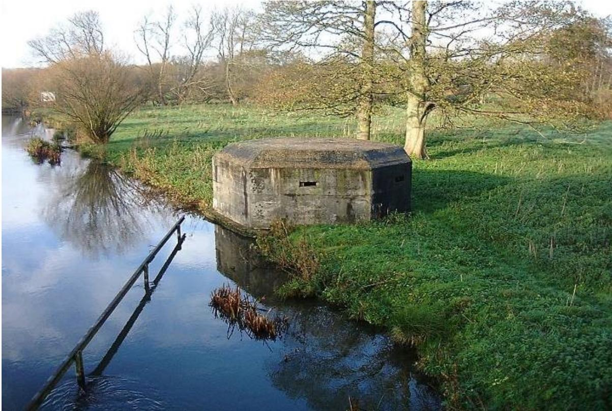
Northcroft pill box is a Type 22 meaning it's small and hexagonal, one of the more common types of pill box. It is believed that the pill boxes built along the Kennet and Avon were built in July 1940. This pill box forms part of the Newbury nodal point. The defences were developed as a nodal point because Newbury was considered an important centre of regional road communications. During 1941 it was reclassified as a Category B anti-tank island.
